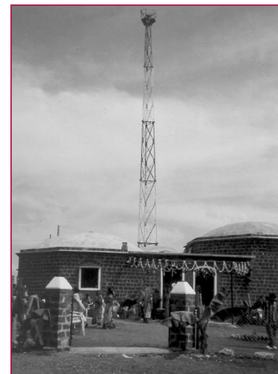
The Pastapur community in India built their own radio studio using locally fired clay bricks. The tower is a professionally fitted self-standing mast with an omni-directional antenna crafted under the guidance of a professional broadcasting technician. Adjacent are five school rooms for 'learning without frontiers' also built from the same kind of bricks.
